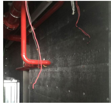
Installation of a soundproofing system
