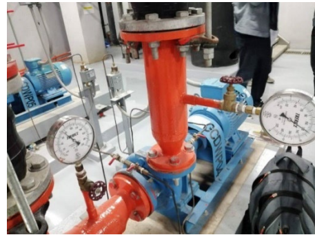
Installation of water pumping system
