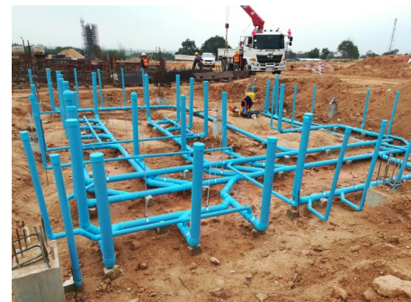
Installation of sewage system
