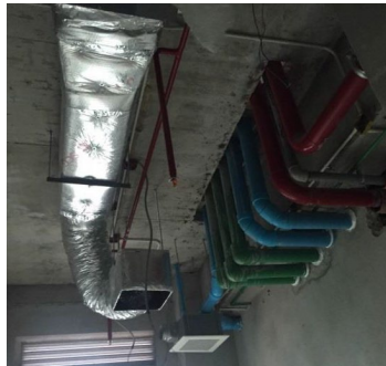
Installation of ducts and cold air outlets
