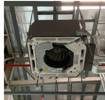
Installation of a small air compressor
