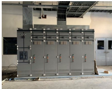
Low voltage electrical system installation (400 volts)
