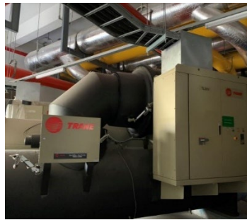
Installation of large air conditioners
