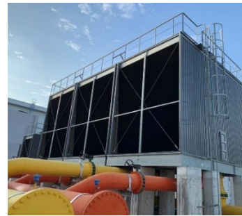
Installation of cooling tower
