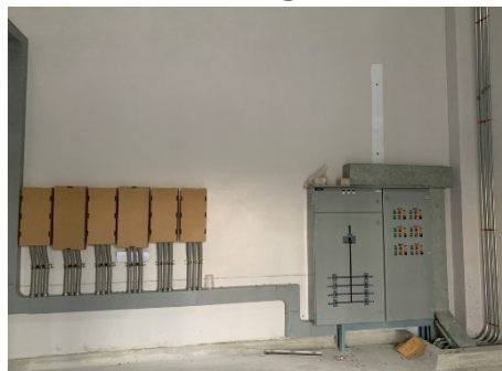
Installation of a water pump control cabinet
