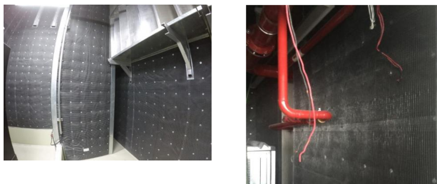
Installation of a soundproofing system
