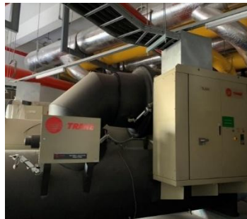
Installation of large air conditioners
