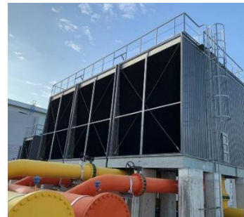
Installation of cooling tower
