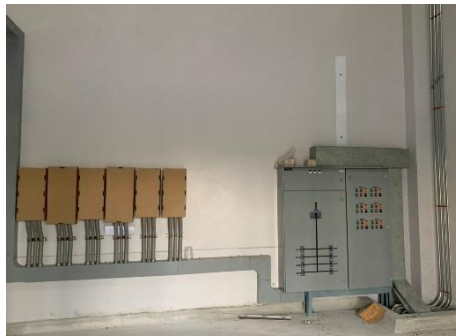
Installation of a water pump control cabinet
