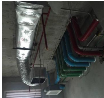
Installation of ducts and cold air outlets
