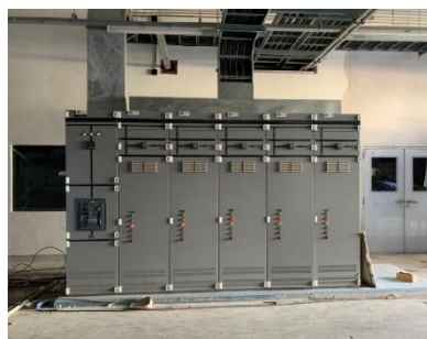
Low voltage electrical system installation (400 volts)
