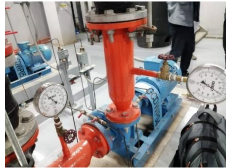
Installation of water pumping system
