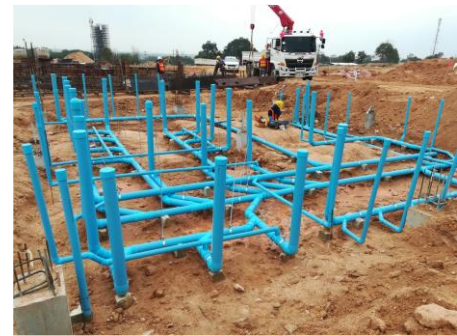
Installation of sewage system
