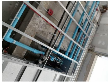
Installation of water pipe systems in buildings
