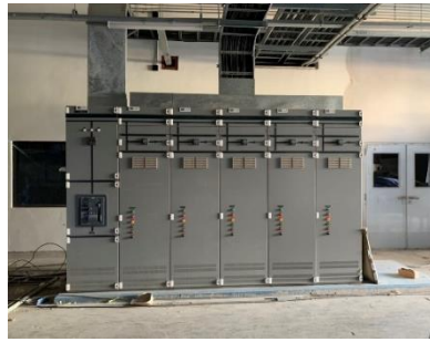
Low voltage electrical system installation (400 volts)
