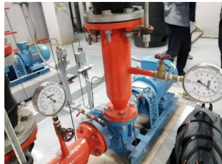
Installation of water pumping system
