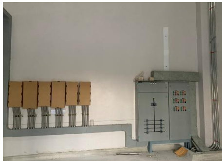
Installation of a water pump control cabinet
