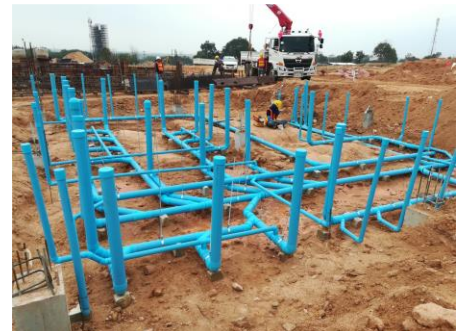
Installation of sewage system
