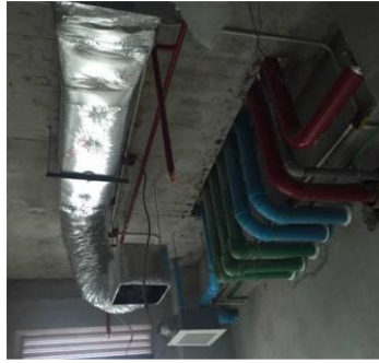
Installation of ducts and cold air outlets
