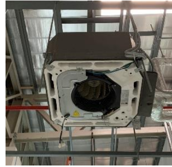
Installation of a small air compressor
