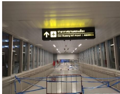
Road sign installation
