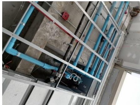
Installation of water pipe systems in buildings
